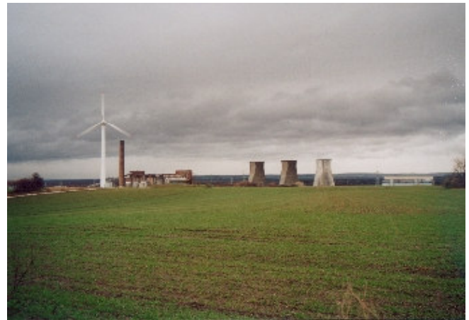
Fig. 7.: Wind, coal and gas turbine plant at Inota.
