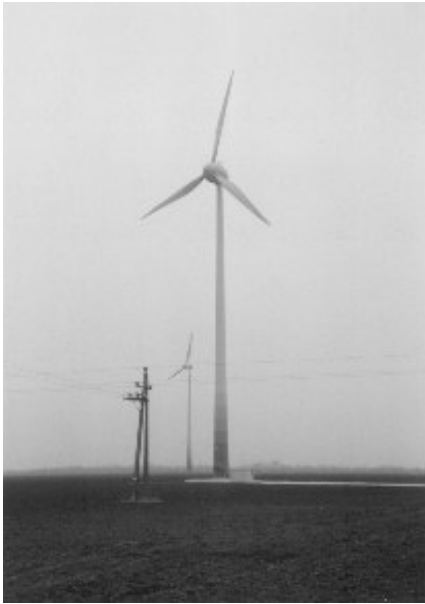
Fig.5.: New wind turbines at Mosonszolnok
